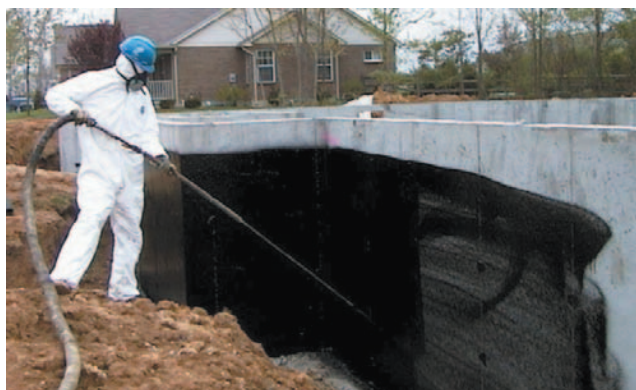
A basement stays dry with J-Cote™ by forming a seamless barrier that stops water even if the basement cracks.
